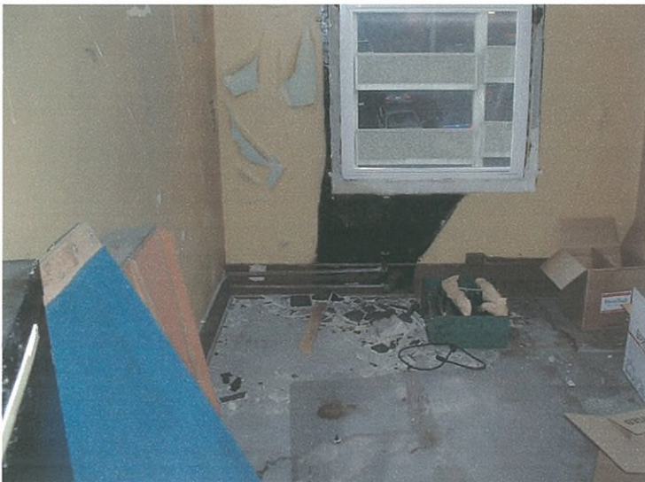
Damaged Plaster in a Sleeping Room
